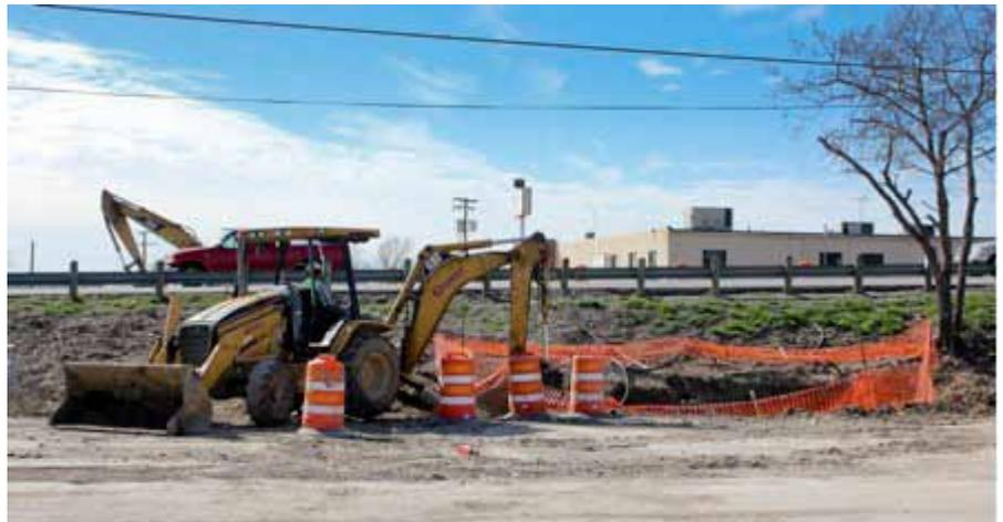
**Fort Worth based Conatser Construction is busy relocating water and sanitary sewer lines for the City of Fort Worth in preparation for Henderson Street Bridge Construction.**
