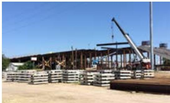
The bridge contractor is currently erecting bridge superstructure falsework on the White Settlement bridge so that the box girders and concrete deck can be constructed. The bridge contractor is currently working on the east and west portions of the bridge simultaneously. Once the falsework is
