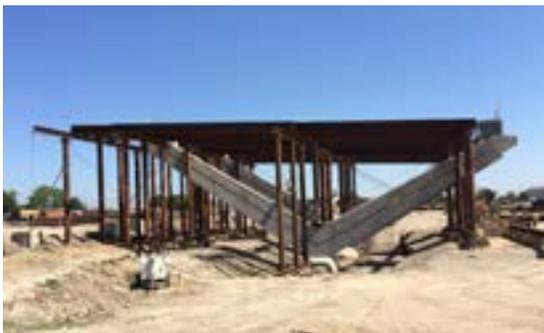
Bent 5 falsework being installed at White Settlement
